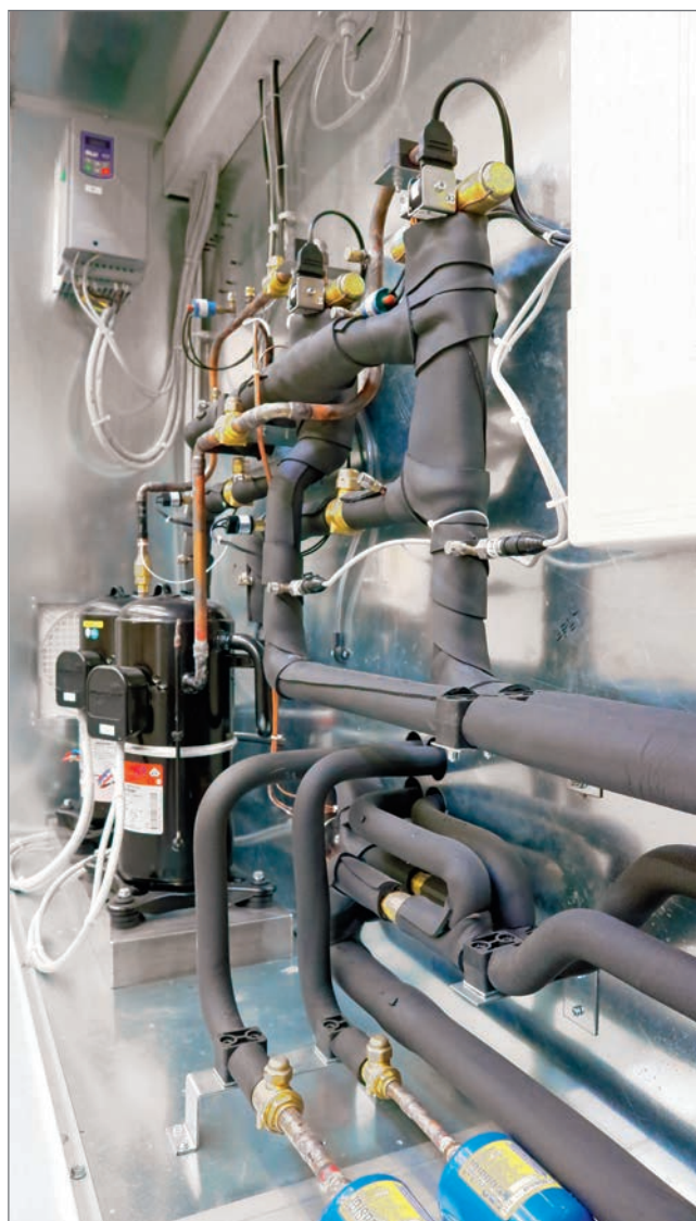
REFRIGERATION CIRCUIT
